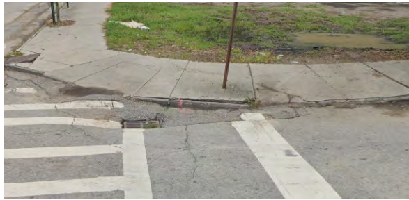
Existing storm drain inlets on the travel lane.
