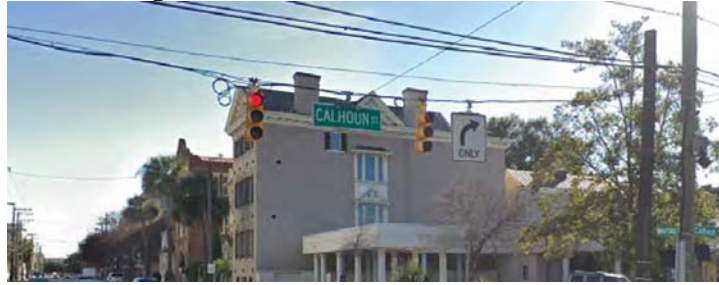
Existing Calhoun St. signal heads without retroreflective backplates.
