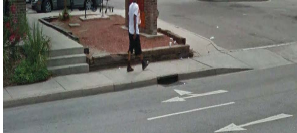
Existing storm drain inlets on the travel lane.
