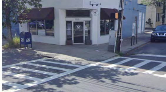
Sidewalk without detectable warning surface at Smith St.
