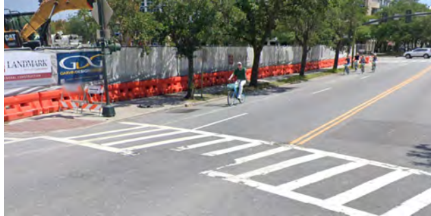
Existing pavement markings worn out
