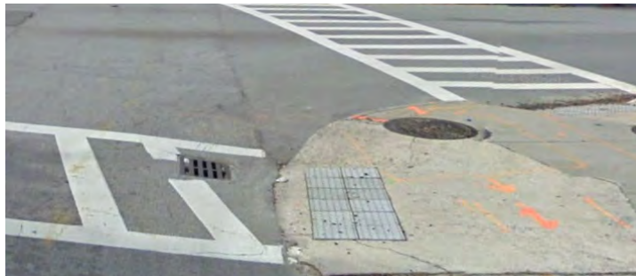
Existing storm drain inlets on the travel lane.
