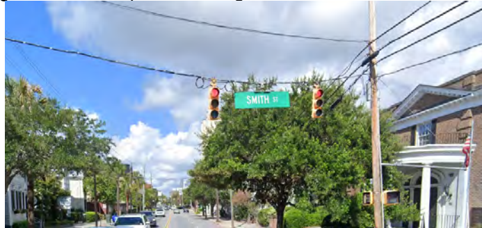
Existing Smith St. signal heads without retroreflective backplates.
